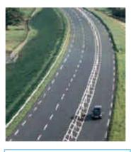
2 Plus 1 Road – A positive measure towards safer motoring
